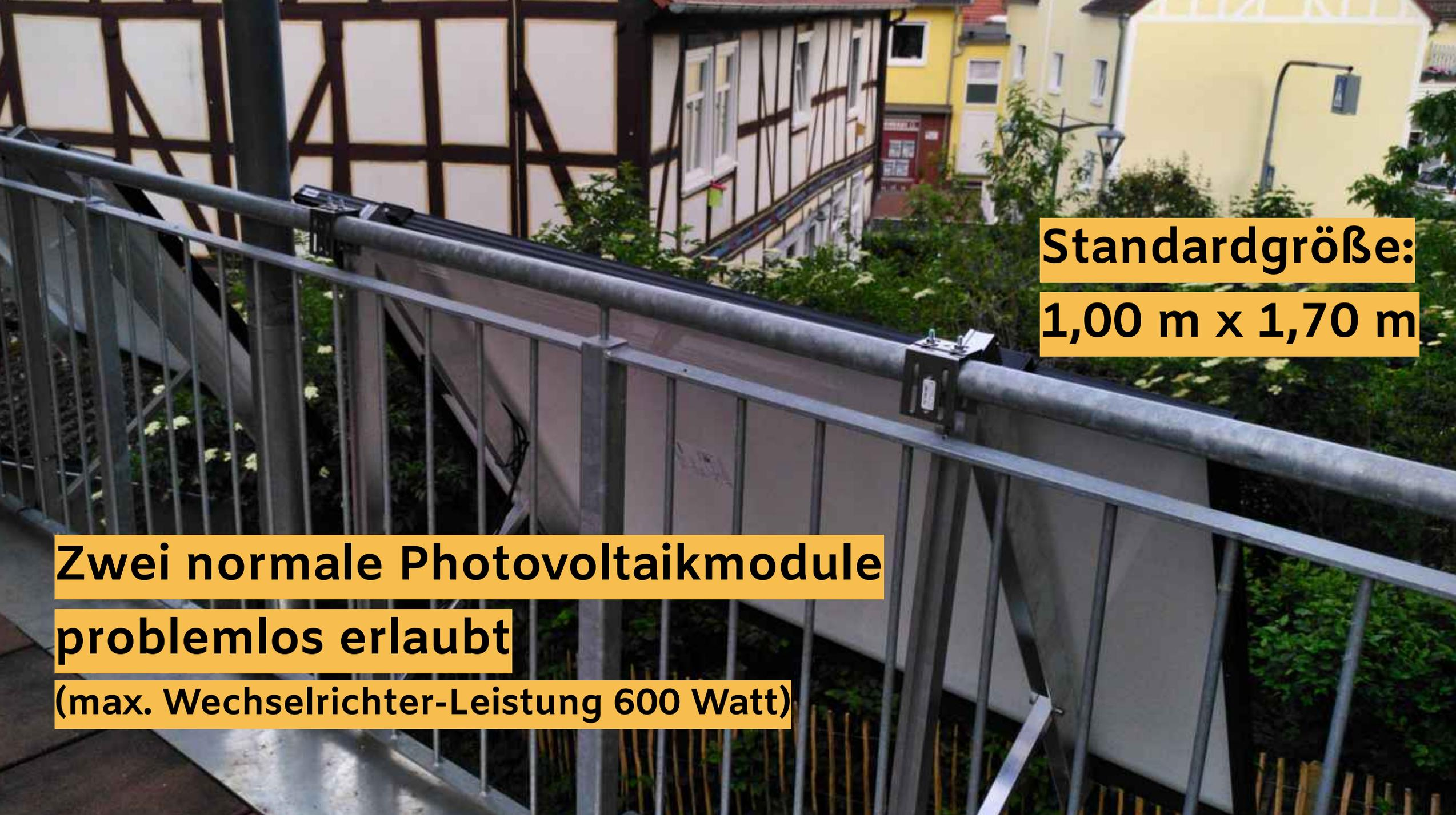
The image shows a balcony railing with two photovoltaic modules mounted on it. The railing is made of metal and has a glass panel. The modules are connected to the railing using brackets. In the background, there are residential buildings, including a half-timbered house and a yellow building. The scene is outdoors with some greenery.
